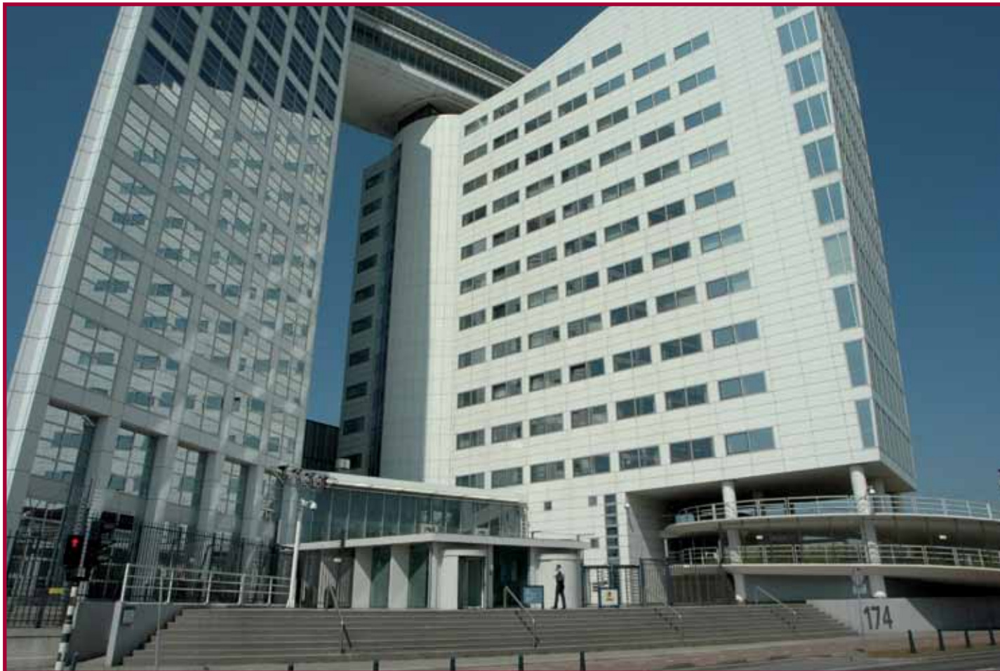
Eurojust Arc building
