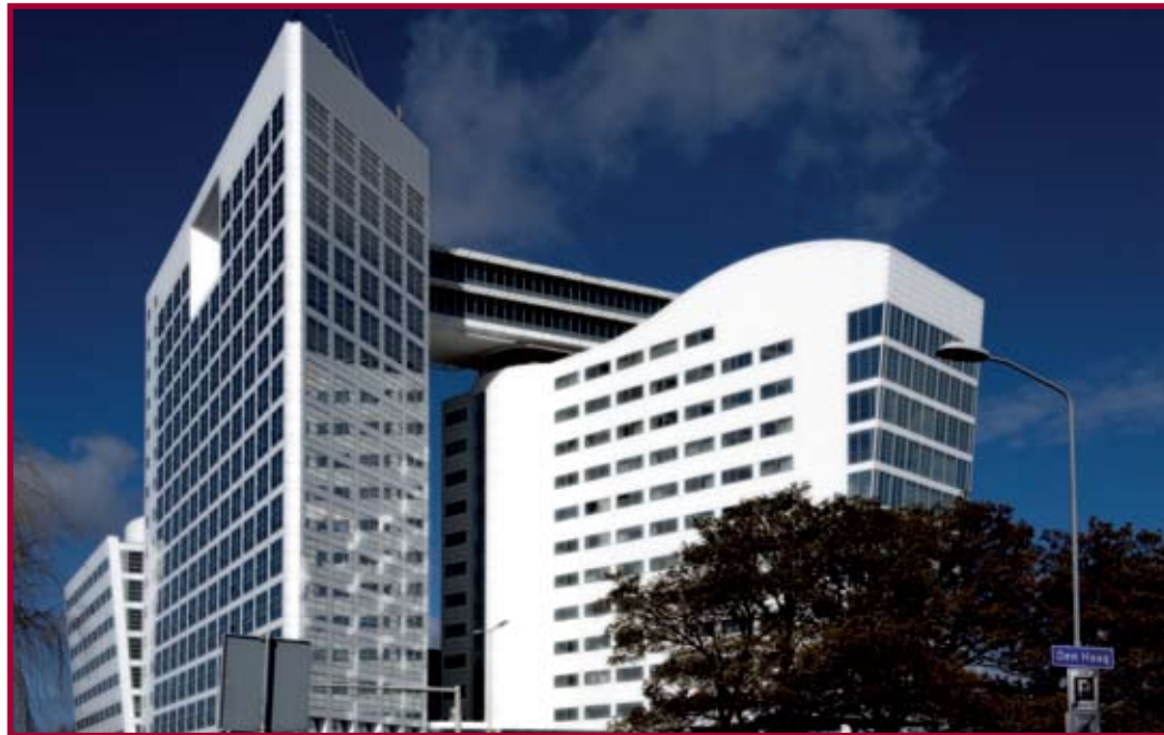
Eurojust building 1 - the Arc
